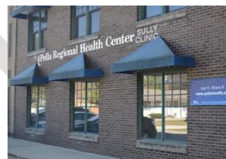
Source: Pella Regional Health Center
