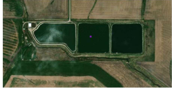
Aerial photo of the Sully wastewater treatment facility. Source: Iowa Department of Natural Resources Facility Explorer
